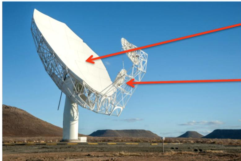
The antenna consists of the main reflector (effective diameter 13.5 m) plus the sub-reflector (diameter 3.8 m). The main reflector is made up of 40 panels, made of aluminum. The sub-reflector is a single composite structure.
