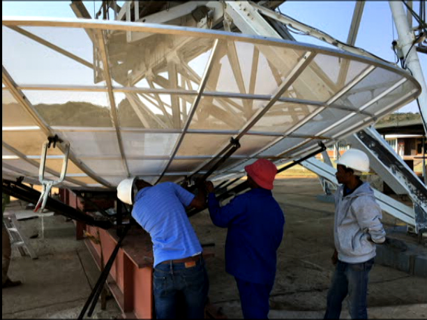
HartRAO technician Andrew Masiteng, UKZN PhD student Onkabetse Sengate and UKZN MSc student Kabelo Kesebonye assemble 6m dish
