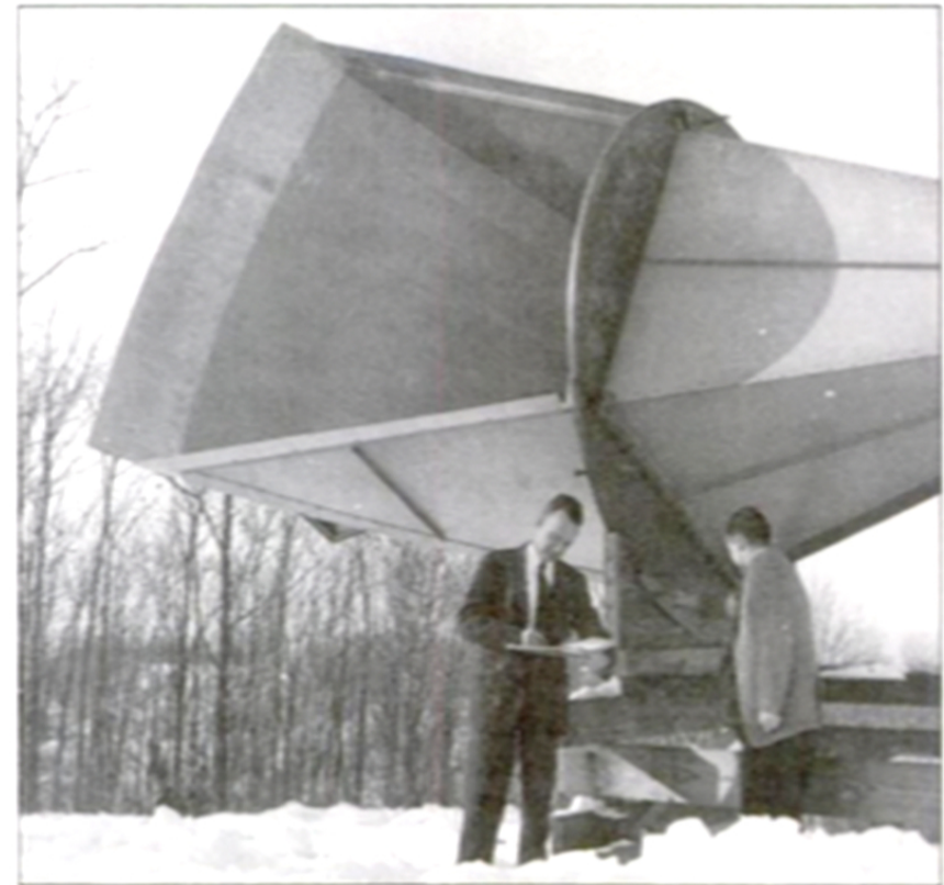
Edward Ohm (right) at the 20-foot horn antenna at Holmdel, New Jersey. He had noticed as early as 1961 that the horn was registering more static than expected when pointed at the sky but had not realized its significance.
