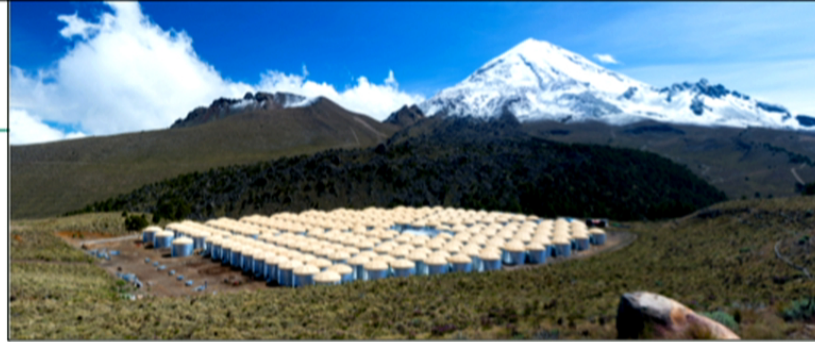
Last Tank Constructed Dec. 2014
