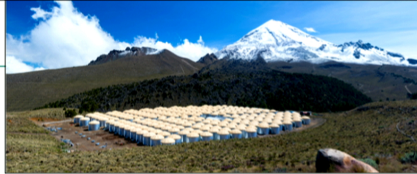
Last Tank Constructed Dec. 2014
