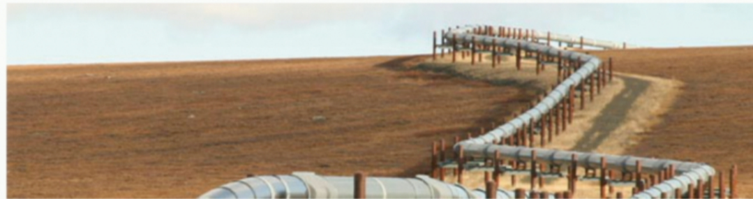
Trans-Alaska Pipeline System
