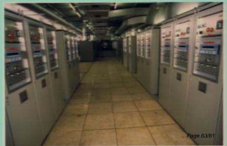
Power supplies for Transfer Line made by Inverpower Controls, Burlington, ON
